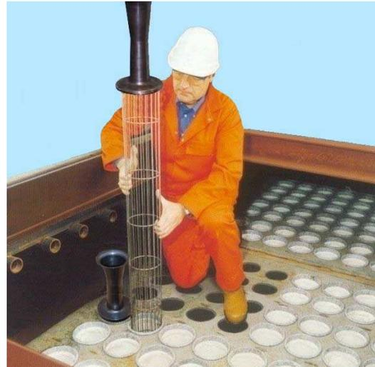
Figure 10 Cage Installation
